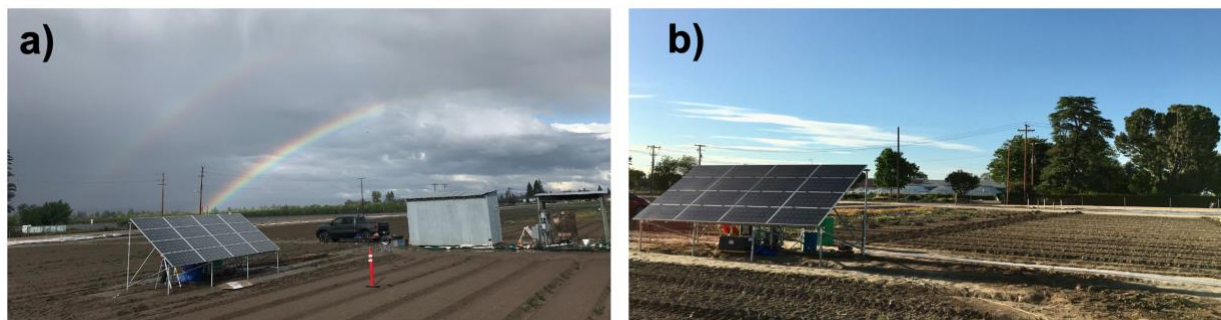
Fig. 1. Two photographs of the on-site solar-fertilizer generator with the 5-ft wide, 40-ft long tomato beds visible in the background. The nitric acid generator is positioned underneath the 3-kW solar array. The image in a) was taken before the season in April and b) after the tomatoes were transplanted in May.
